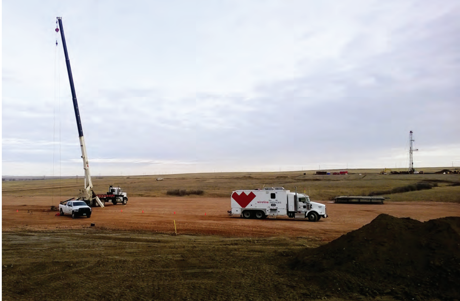
Fig. 3. Weatherford's rigless wireline solutions streamline P&A and gas-lift interventions, reducing cost and complexity without a workover rig.
