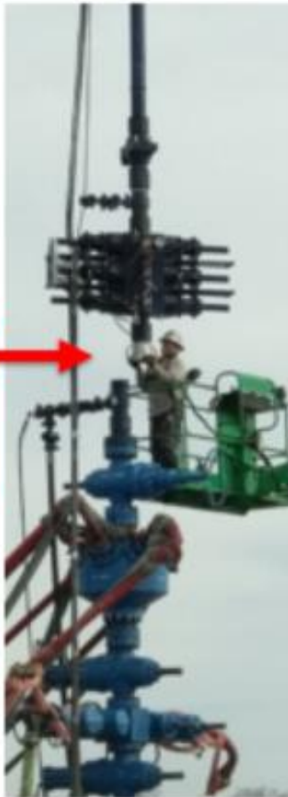
Original Lubricator Connection Method
